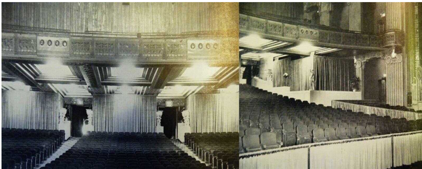
The scheme of seat partitions in the general rear view and the side view. Flood lights in the balcony fascia illuminate the drapery. (Images from the trade magazine "Motion Picture Herald" dated 03.12.1960)
